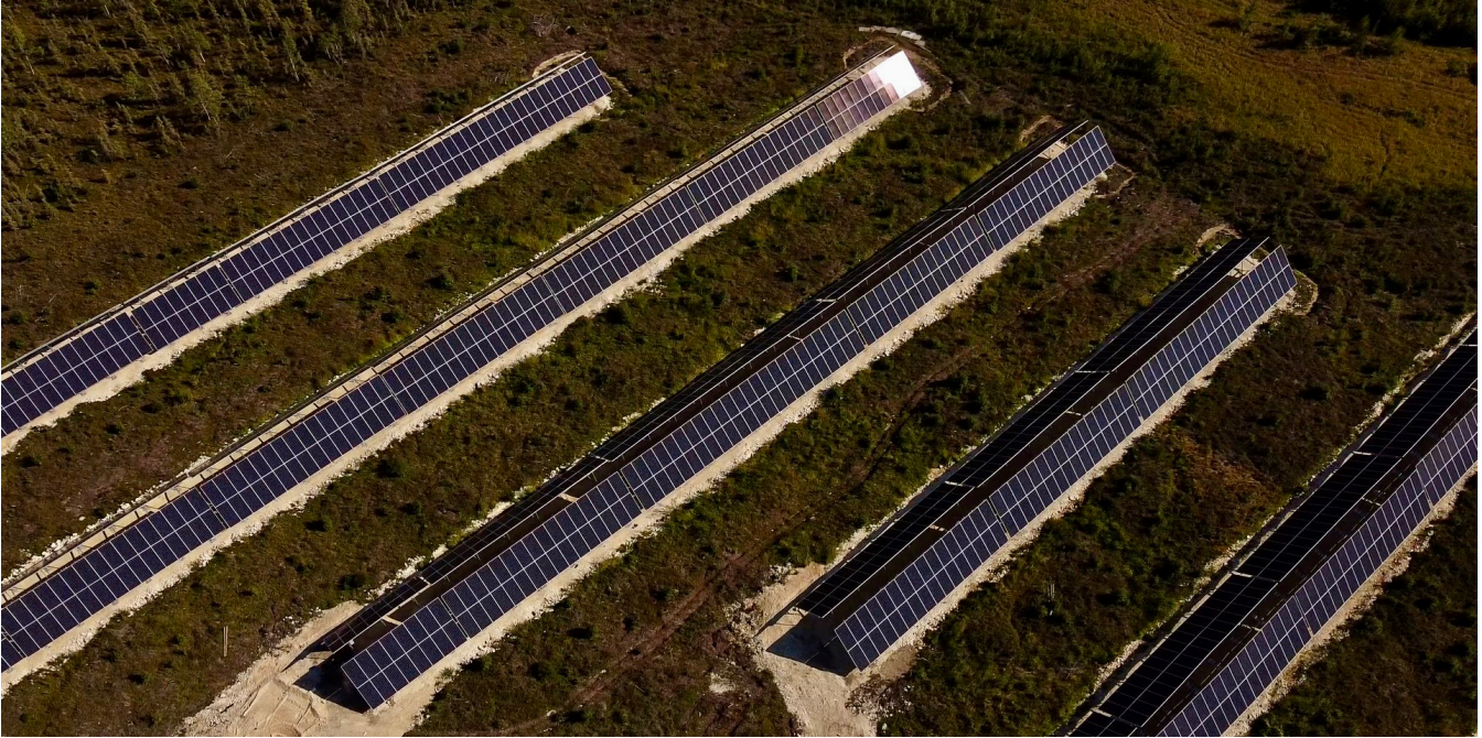
An aerial view of Sree Vyah showing the mono-crystalline panels positioned in an east-west orientation to maximize solar generation during the long daylight hours of the Arctic summer. Photo by Caleb Charlie
